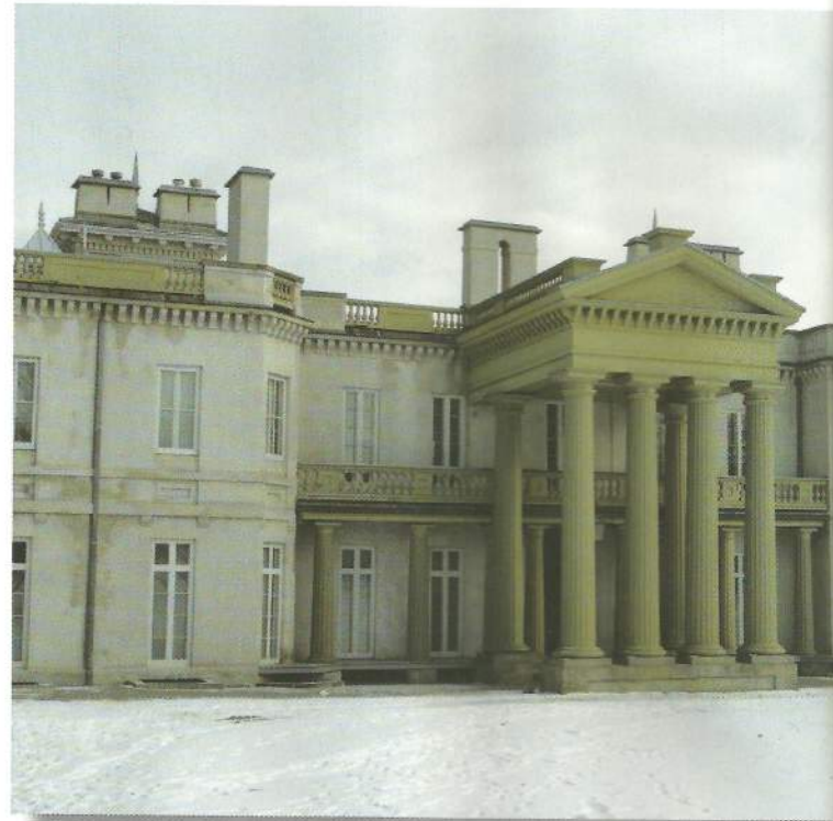
Sir Allan MacNab’s imposing 19th century Regency Italianate mansion crowns Burlington Heights. When you visit the museum, be sure to tour the kitchen garden and outbuildings, as well as the Hamilton Military Museum. Today’s peaceful and gracious grounds were occupied by soldiers during the War of 1812.
